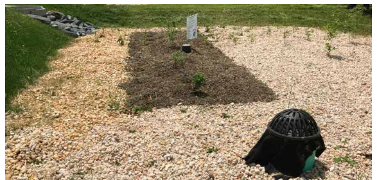
Covered Beehive Overflow filter, gravel and mulch.
