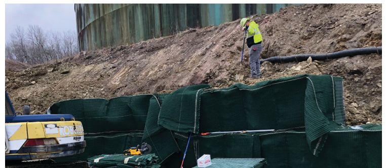
Second layer of Scourlok being covered with soil following being filled (1 cell deep).
