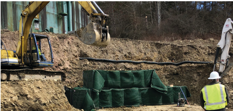
Machinery filling cells with on-site material.
