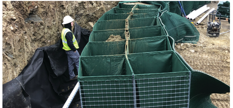
Scourlok flexibility to work with radial alignment.
