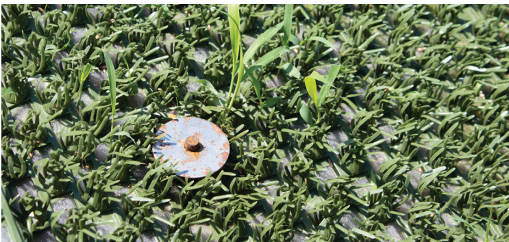
Anchored using pins and washers.
