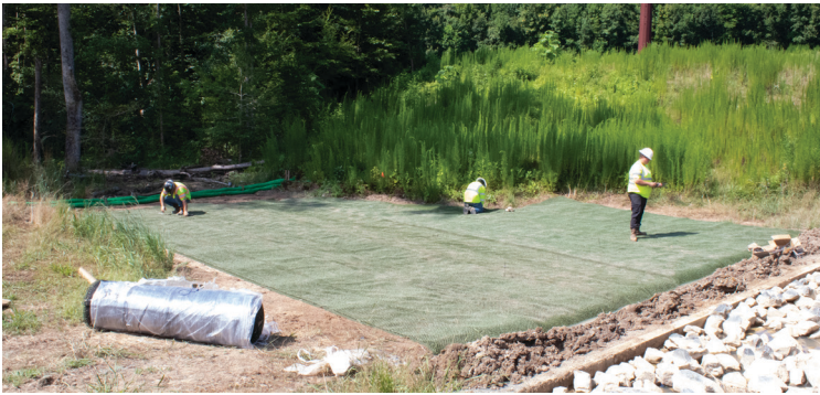
Before hurricane—emergency spillway.
