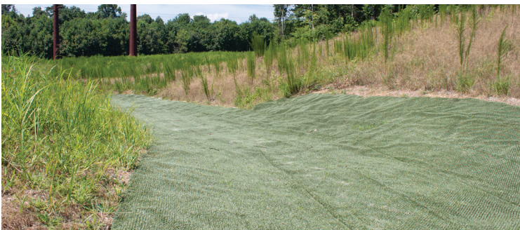
Before hurricane—outfall channel.
