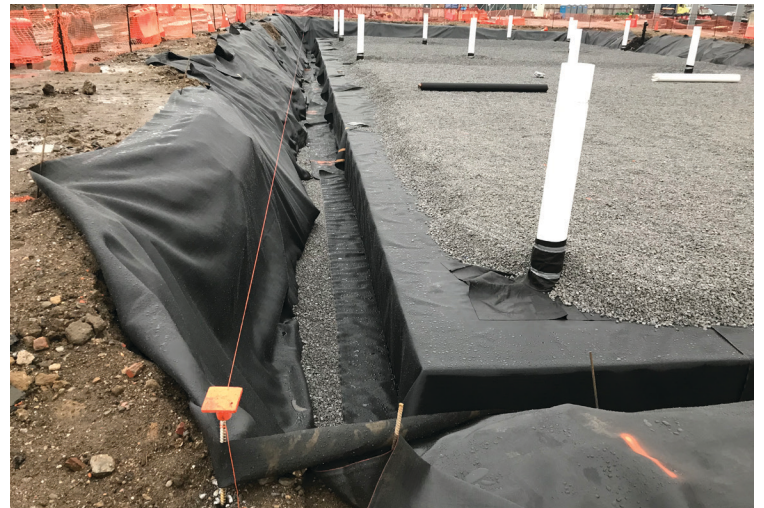
Side backfill and geotextile wrap.
