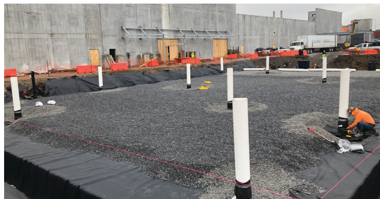
Stone backfill and maintenance ports.
