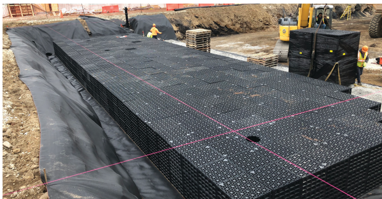
Placement of R-Tank UD modules.
