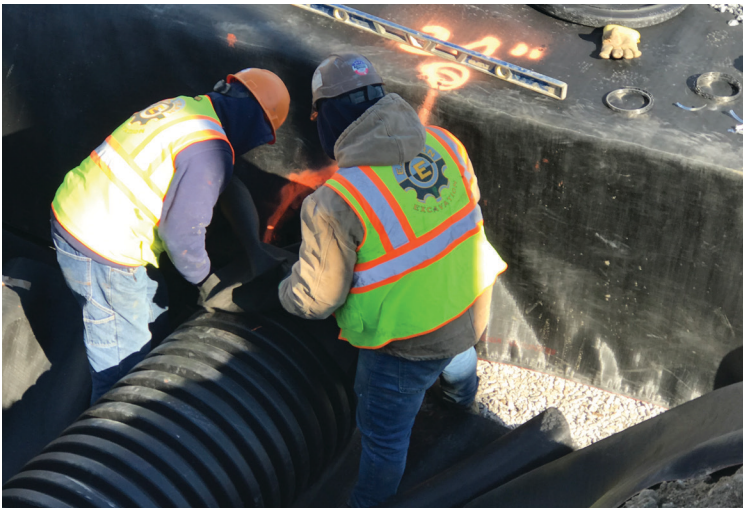
Connection of pipes with geotextile boot kits.
