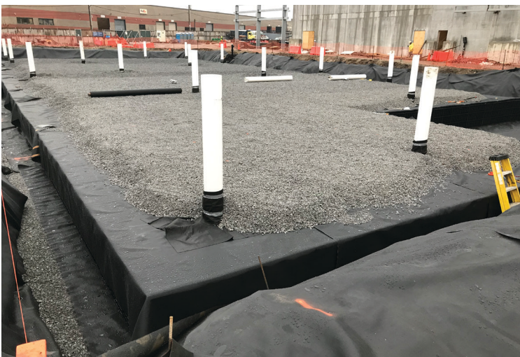
Progress of initial 12-in stone cover.
