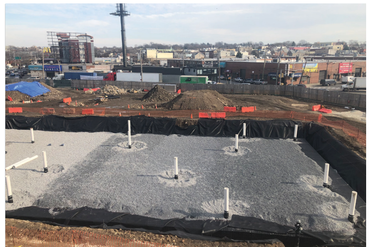
Progress of initial 12-in stone cover.
