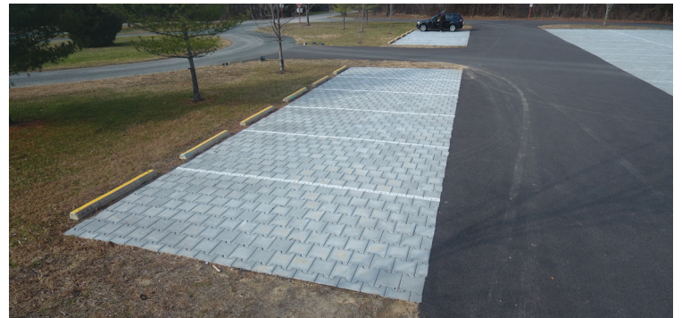
Asphalt drive aisle paired with PowerBLOCK.
