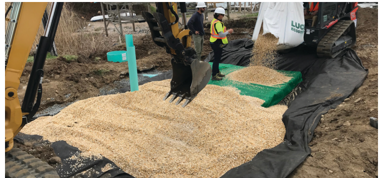
Microgrid mesh installed, then the top and sides backfilled with peagravel.
