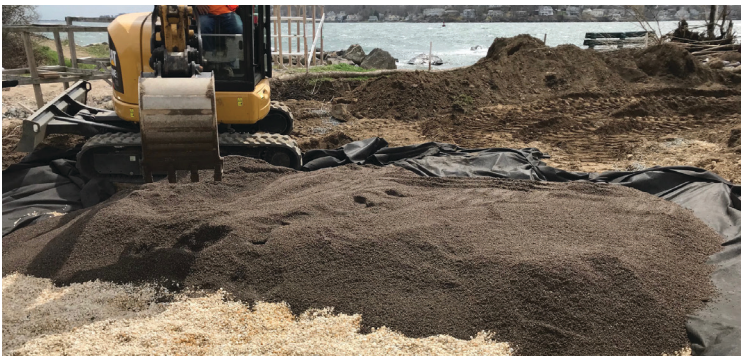
High performance biofiltration soil installed.
