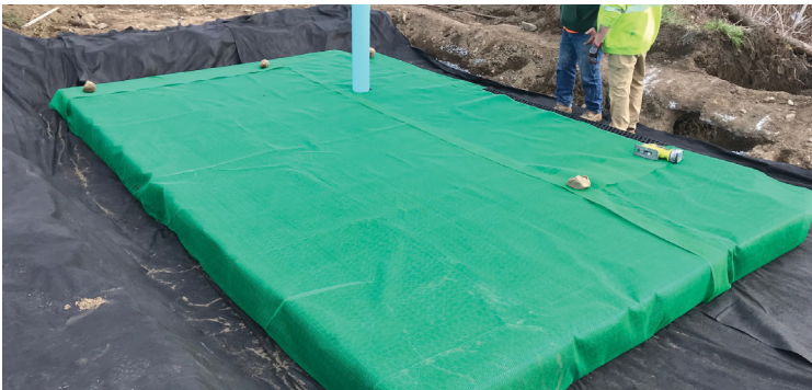
Modular underdrain installed inside geotextile envelope along with the maintenance port.
