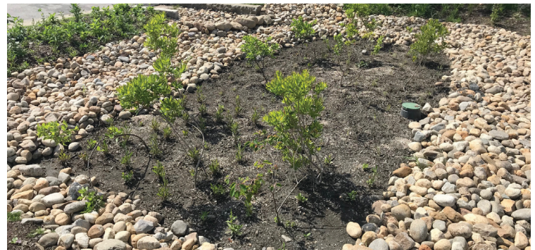
Plants, mulch and rocks top off the biofiltration system.
