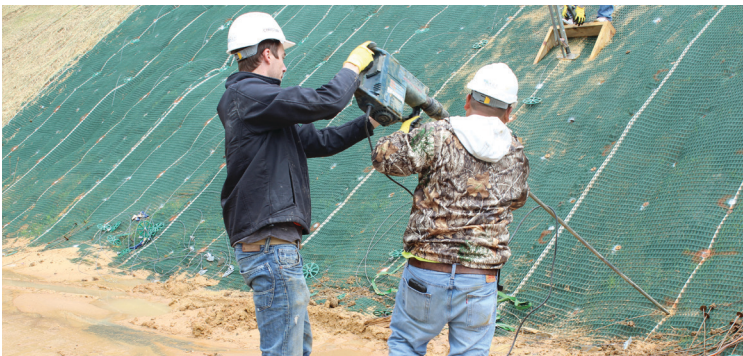
Engineered Earth Anchors installation using a power driver.
