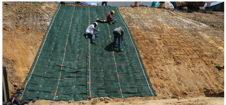
Beginning of Armormax install with Pyramat rolled down the hill and washer pins installed.
