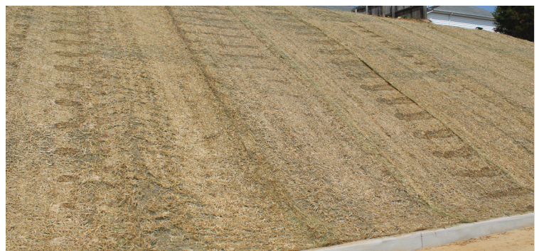
To protect the installation and new vegetation, a straw erosion control mat was installed.
