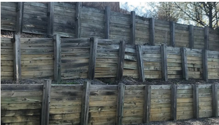
Prior to installation—bowing wall
