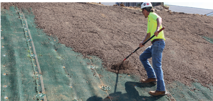
To promote vegetation, seed was placed beneath Armormax, beneath evenly spread soil coating and above soil coating.
