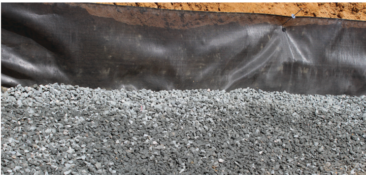
Installation of trench drain using geosynthetic fabric to protect from seepage.
